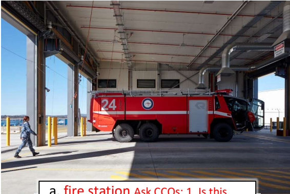
a. fire station Ask CCQs: 1. Is this where fire trucks stay? (y); 2. Can you see a fire station only at an air force base? (n, you can see them in many places e.g. cities, airports).
